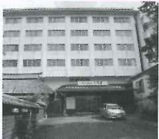
▲旧ホテル関所解体前
